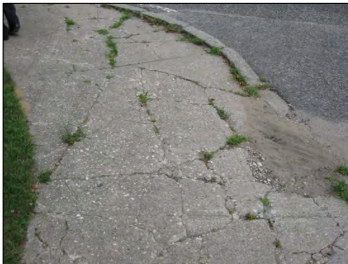
Photograph No. 4: View of deteriorated sidewalk/curb area at Union Avenue and Mill Road.
