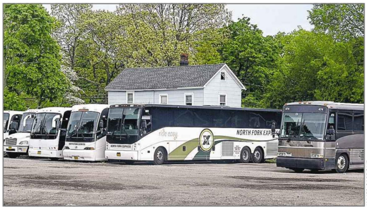
The North Fork Express charter bus depot occupies a 2.2-acre lot on Hawkins Avenue.
